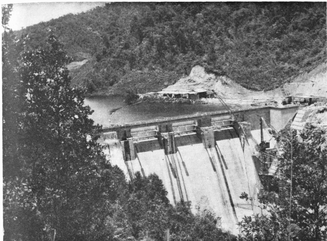
FIG. 4. Construction of the Ringlet reservoir dam, part of the first stage of the Cameron Highlands scheme. Water from the 1.48 million cubic feet reservoir reaches the underground Jor power station, 1,900 feet below, through several miles of tunnels. (CEB photograph).
